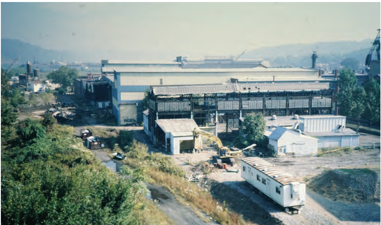
Pictured: The NREC facility in the early stages of demolition/renovation in 1995.
